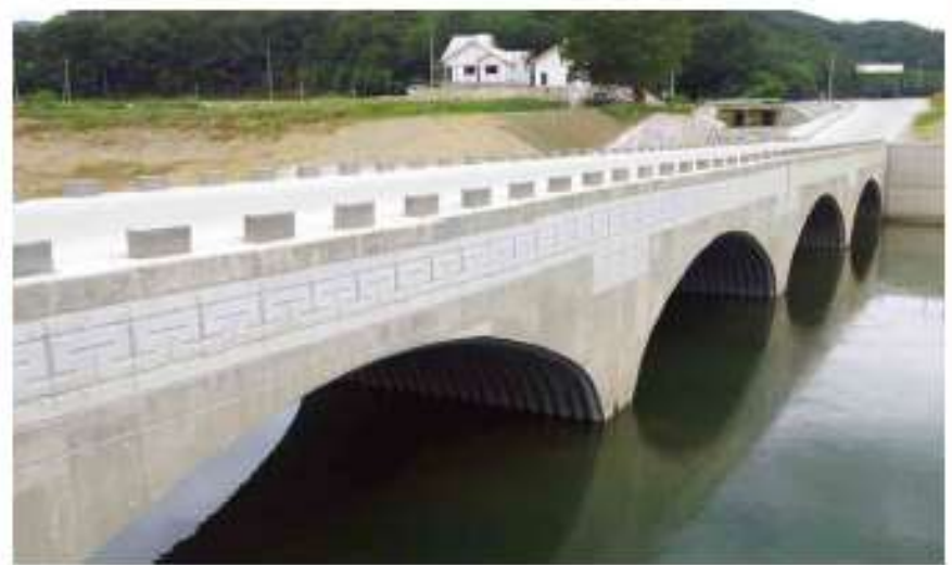
Namsan Boori Hill (Good/2012) | Type : Low profile arch / Span : 17.0m / Rise : 5.2m / Length : 18.6m
