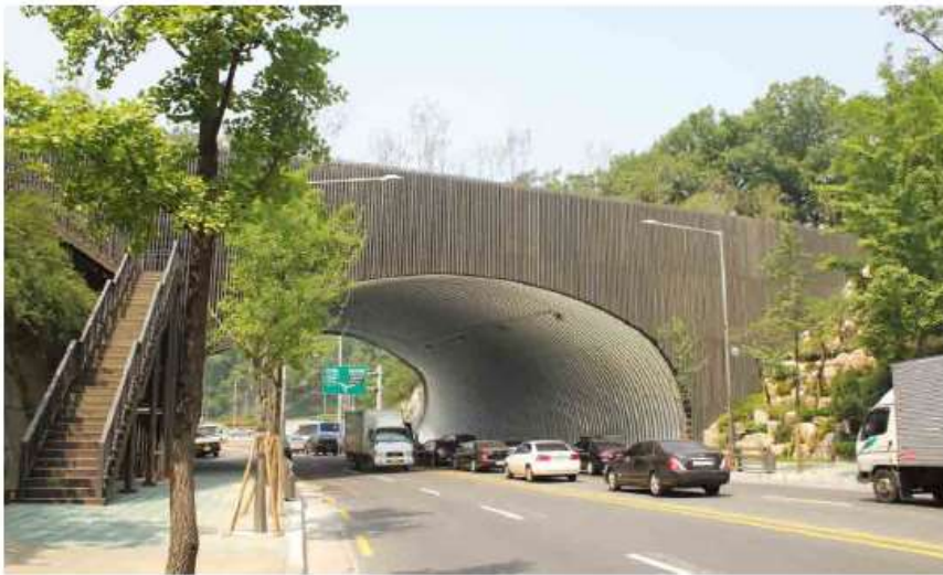
Namsan Boori Hill (Good/2012) | Type : Low profile arch / Span : 25.5m / Rise : 9.1m / Length : 42.6m
